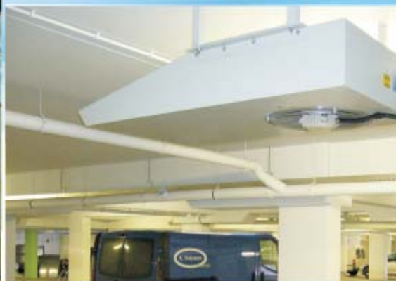
Figures 14(b). Typical JetVent fan installations
