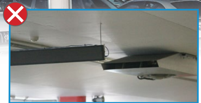
Signs can impede fan throw
